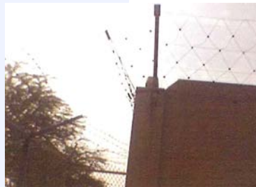
Installed on concrete walls
