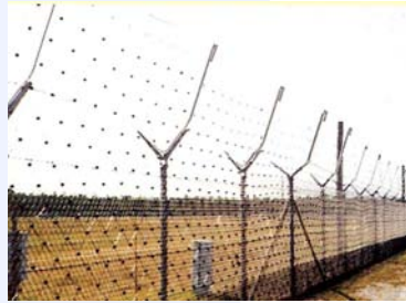
Attached to conventional fencing
